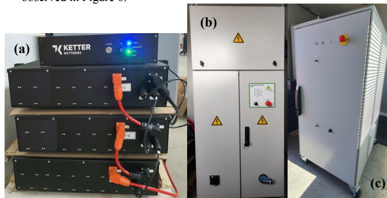
Fig. 6 (a) NMC Battery. Fig. 6 (b) DC/AC inverter. Fig. 6 (c) DC/DC converter. Own source.
