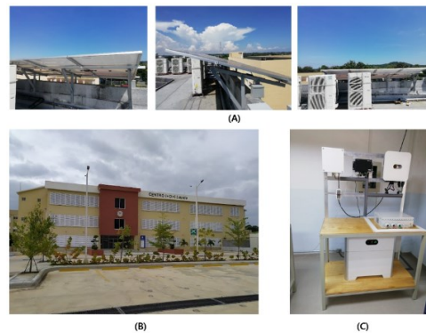
Fig. 4. Front view of CIDIL, where the 2.20 kWp PVS is located, Lat. 18.41^{\circ} y Long. -70.1^{\circ} .
